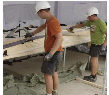
The end of each section has finger-joints which are connected on site, with a glulam wedge glued underneath the intersection for support and to deal with beam tension. Special chain clamps are used to pull the different elements together. The glue technology was developed and patented by Hess.
