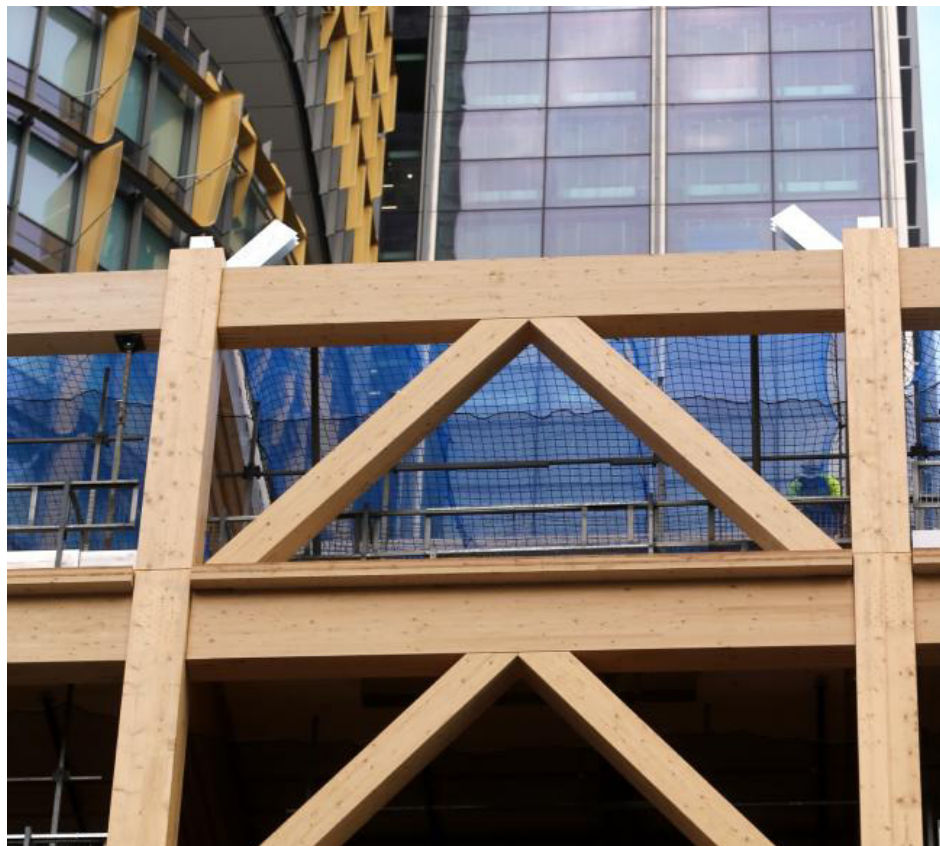
📷 The wooden frame is manufactured in a factory before being brought to the site. Picture: John Grainger
