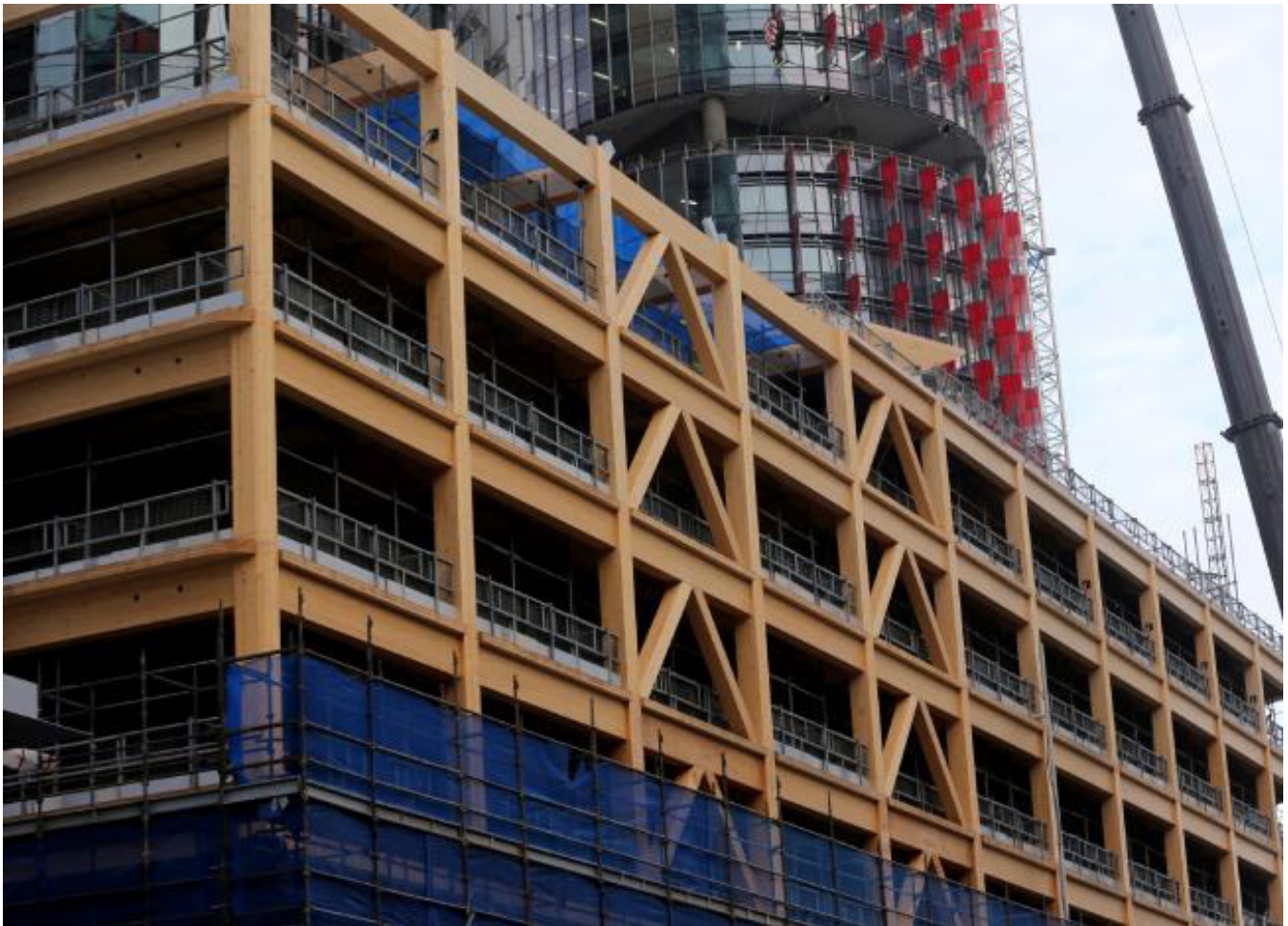
📷 The wooden frame is manufactured in a factory before being brought to the site. Picture: John Grainger
