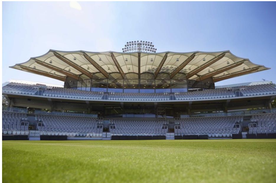
The American white oak glulam beams take centre stage at the new Warner Stand at Lords Cricket ground.
