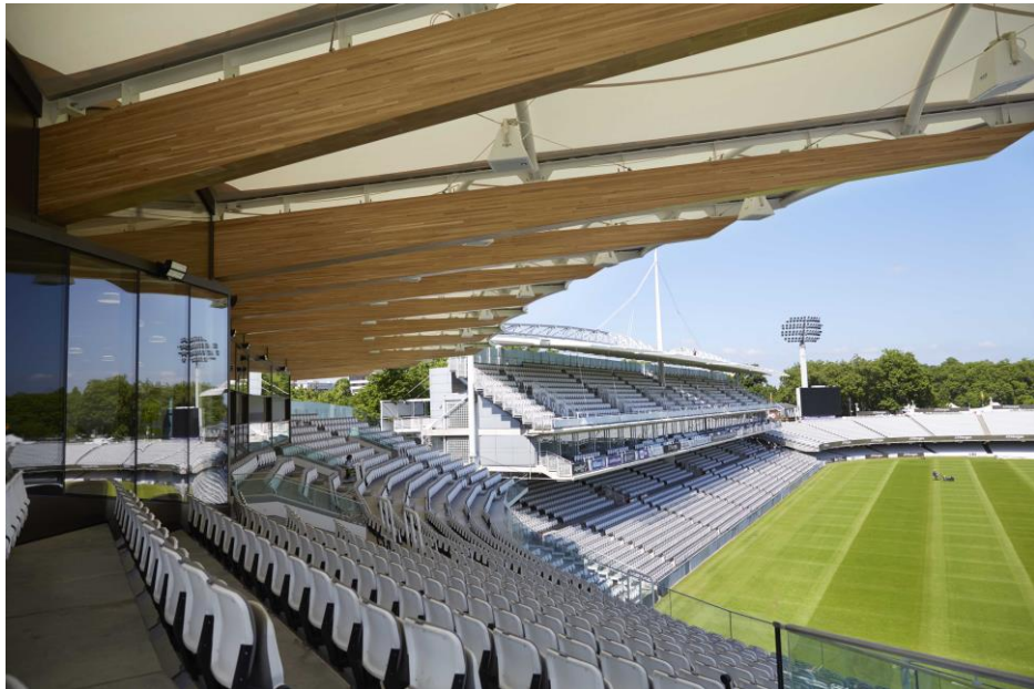
The 23.4 metre long glulam beams stretch across the stand, providing shelter for the guests.
