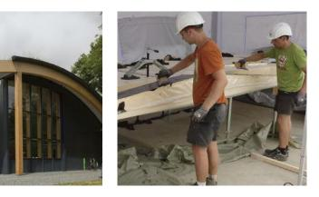
The end of each section has finger-joints which are connected on site, with a glulam wedge glued underneath the intersection for support and to deal with beam tension. Special chain clamps are used to pull the different elements together. The glue technology was developed and patented by Hess.
