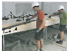
Gluing the wedge member
