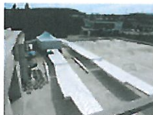
Limitless beams and wedges on site before connection
